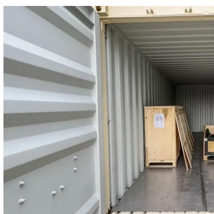
Energy storage container, BESS container
