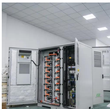
Seplos 50kWh high-voltage energy storage container
